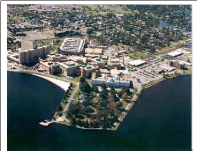
Aerial view of the Naval Hospital.
