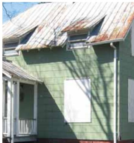
The original wood siding on this vacant house was covered with asbestos shingles which appear to be in good condition.
