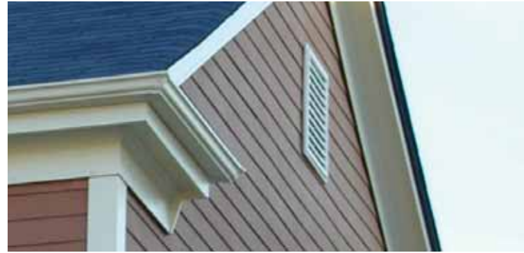
New construction outside of the historic district has successfully used substitute materials, such as cementitious siding and trim details, to achieve a traditional appearance.
