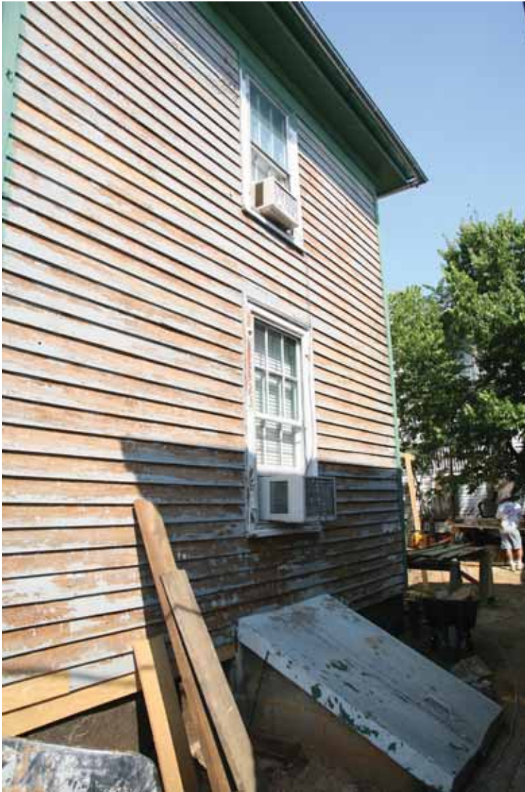
This wooden siding has been sanded to remove all unsound paint and rotted boards have been replaced where necessary. Next step: primer.
