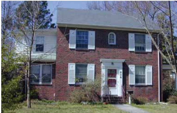
The Colonial Revival style often used brick veneer, a single depth of brick over a wood frame, to make brick a more affordable option for many homeowners.
