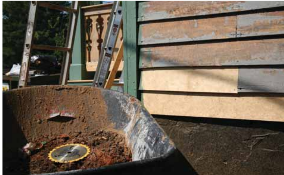
Wood needs consistent maintenance. By keeping siding and trim repaired and painted, you can protect these features from moisture penetration, especially near the foundation.
