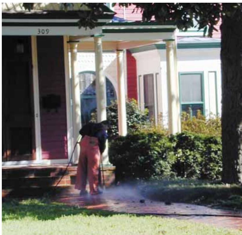
Low-pressure power-washing can be an environmentally sensitive approach to cleaning historic masonry.
