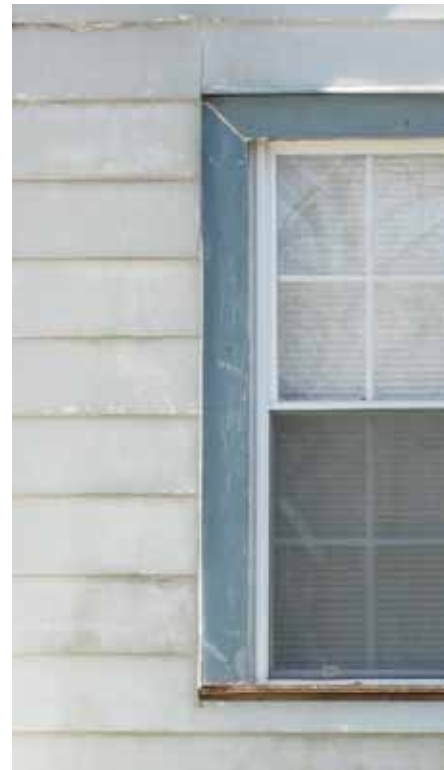
Often, the effects of cleaning or painting vinyl siding can leave the siding with an uneven appearance.
