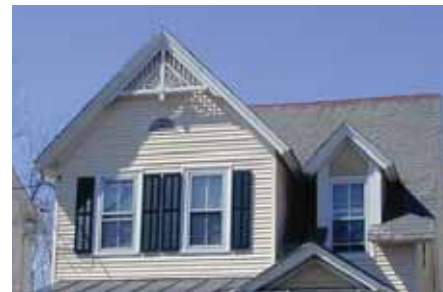
Intricately carved wooden details, called bargeboards, often highlight the apex of an end gable.
