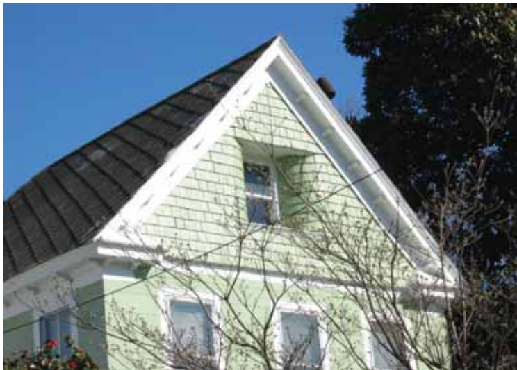
Vernacular Victorian residences also used wood ornamentation as seen in the shingle-clad inset window above.
