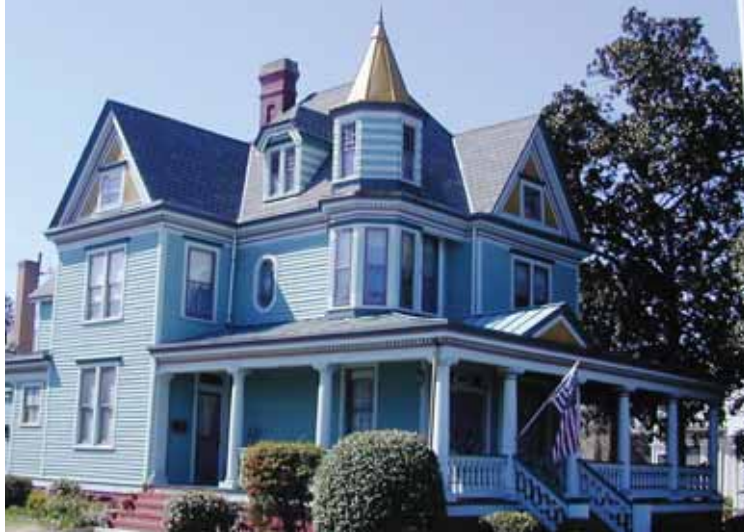
High-style Queen Anne residences used wood ornamentation and texture variations to add interest to the facade.
