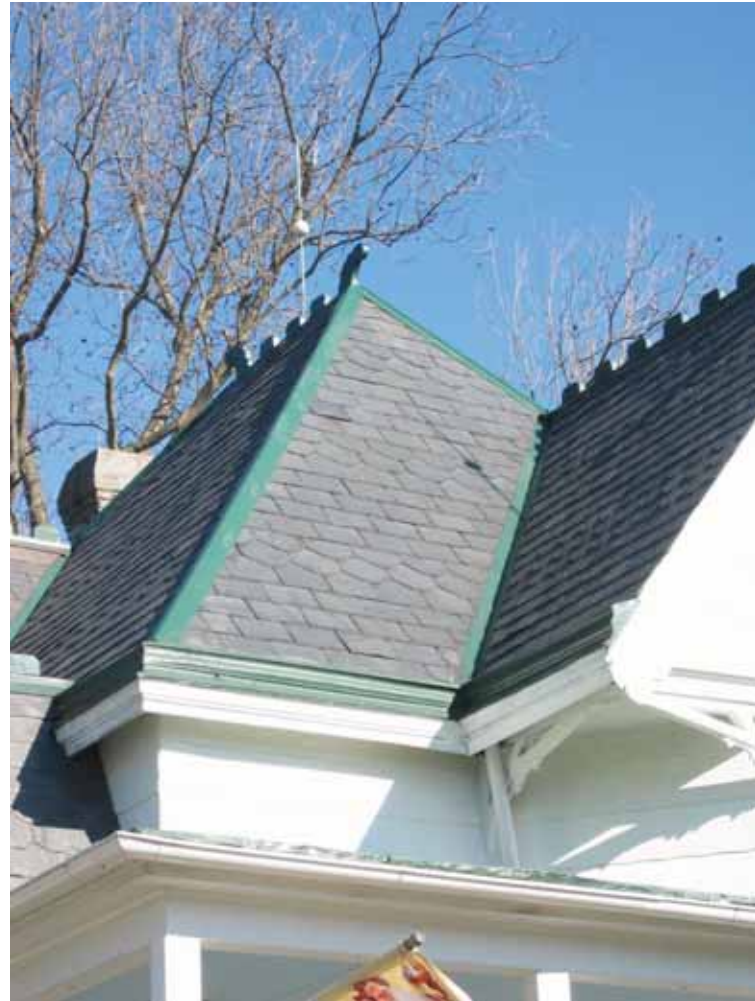
Metal roof cresting often caps the ridgeline of slate roofs in Port Norfolk.
