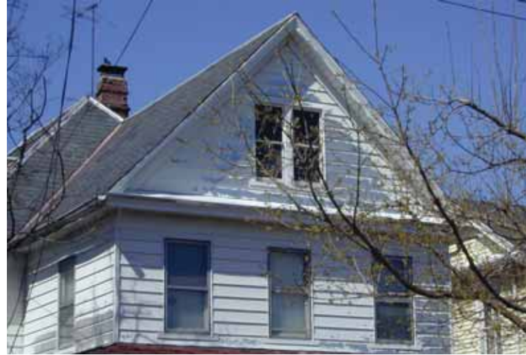
Metal siding may eventually lose its painted coating, exposing the aluminium beneath.
